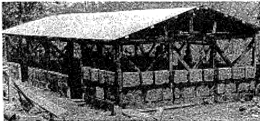
42 Model house built by Oxfam and World Neighbours, using safe construction techniques
