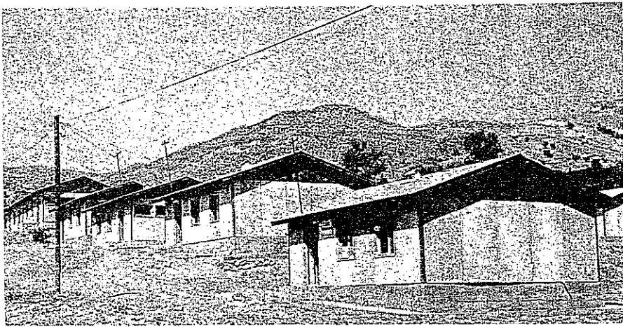
7 New housing in Lice, Turkey, following the earthquake of September 1975
