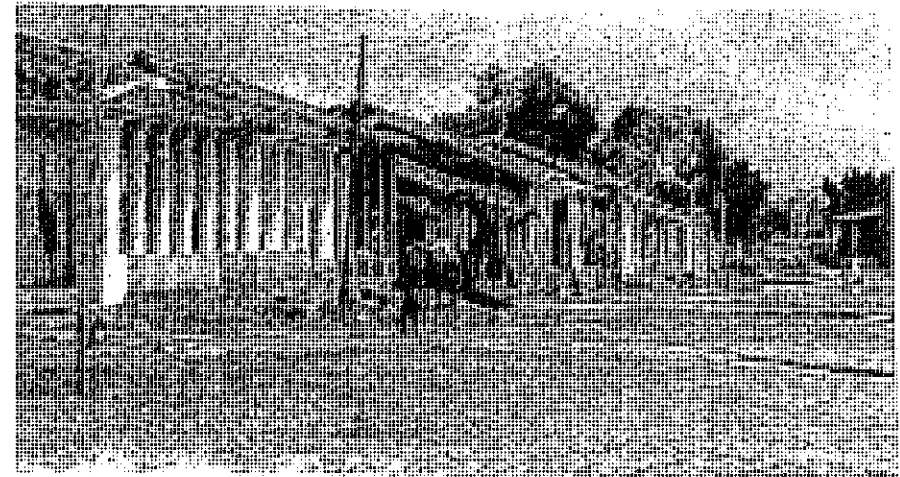
10 Housing in Trinidad, Bolivia, with raised plinths to protect buildings from flooding. In this instance the flooding was so intensive that its level rose above the elevated floor level.
